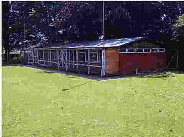
Fig.1 The existing pavilion from the north west.
