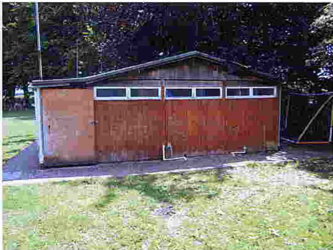
Fig.5 The west elevation of the existing pavilion.
